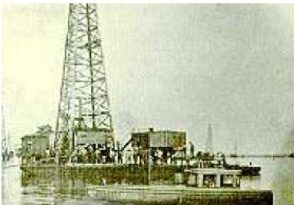
Figura 70 -Balsa com torre de perfuração -Fonte Louisiana Secretary of State of Museums, 2001.
